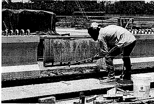
Figure 3.10: Release of Prestress by Flame-Cutting
