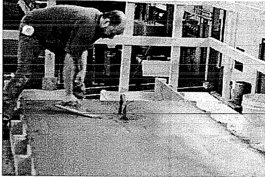
Figure 3.16: Trowel Finishing of the Deck Surface
